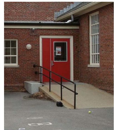
Image 19 Ramp on West Side of building
