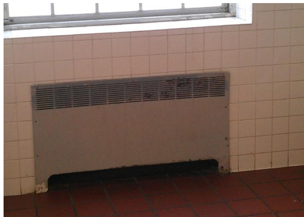
Typical Convector Recessed In Wall
