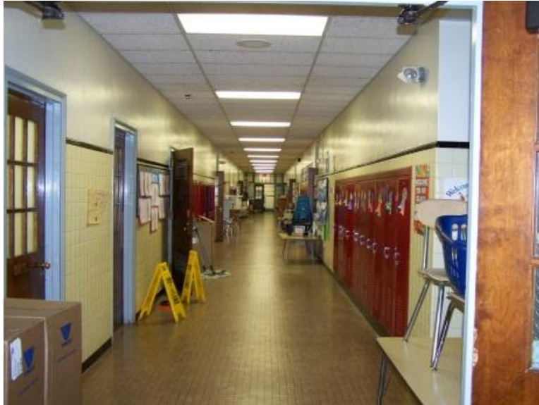
Typical Egress Lighting and Exit Signs
