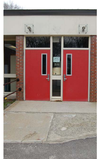
Image 17 Tower Ave Entrance
