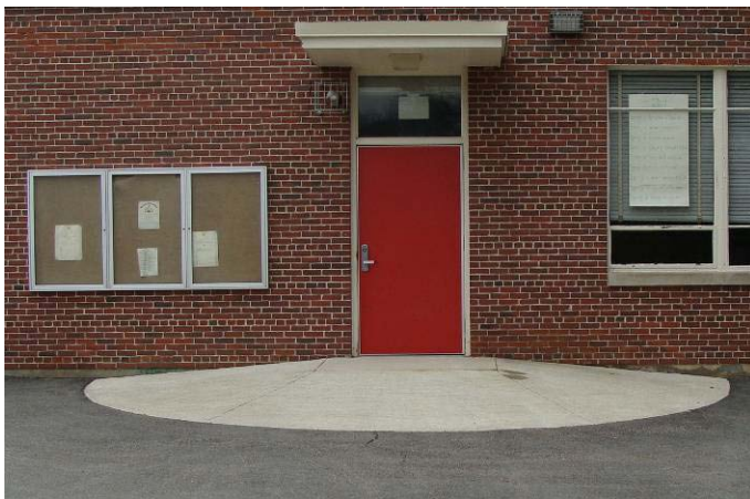
Image 18: Entrance to Kindergarten Rooms
