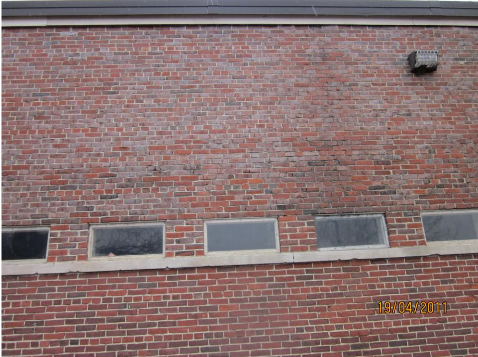
Photo 1: Exterior wall conditions.
